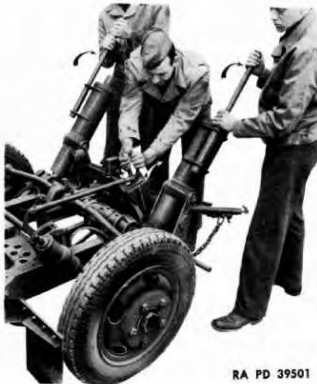
Figure 39 — Lowering Front of Carriage to Firing Position
