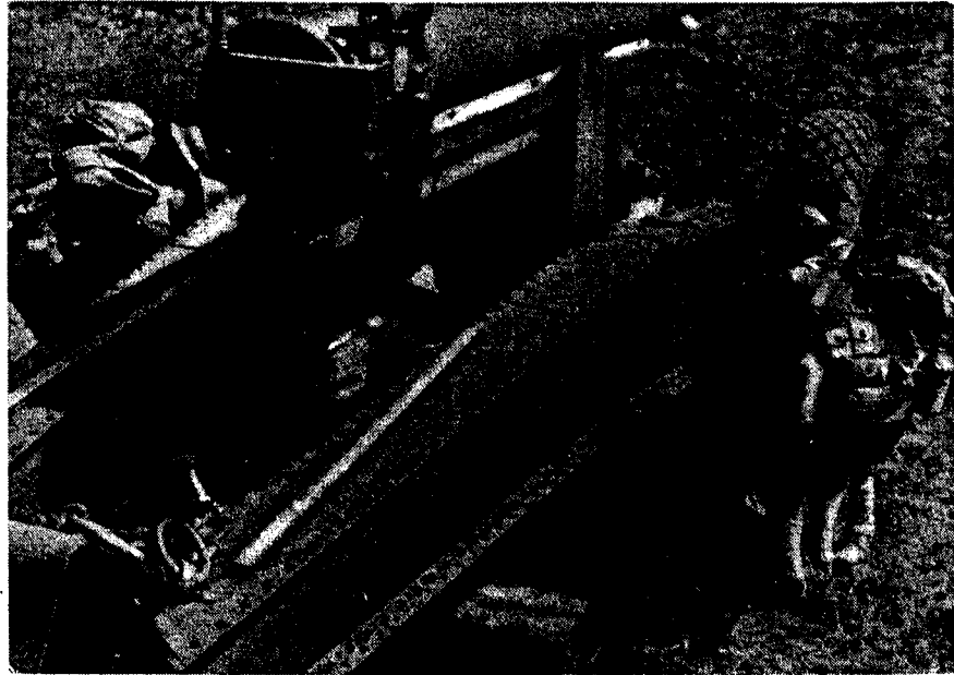
Figure 66—Placing the jack beam under the trails
