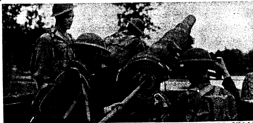
Figure 80—Swabbing the powder chamber
