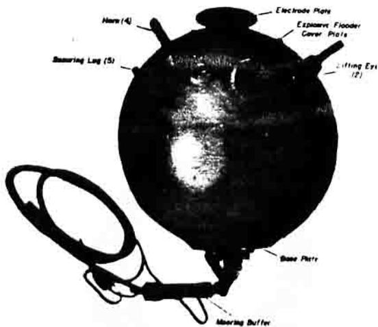
Figure 15 - EMD II Mine - Upper-Lower Antenna
